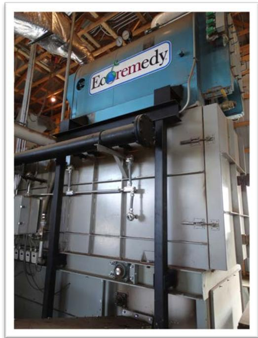
*The Ecoremedy gasifier shown here was installed on Flintrock Farm in Pennsylvania to provide heat to four poultry houses.*
