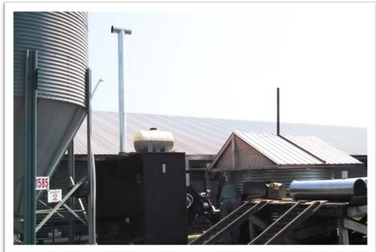
*The Bio-Burner 500 at Riverhill Farm in Virginia was modified to accept poultry litter as a fuel.*
