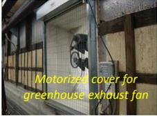
*Motorized cover for greenhouse exhaust fan*
