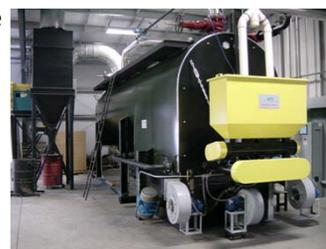
5,000 kW<sub>th</sub> biomass boiler (efficient combustion made possible by new designs and advanced electronic controls)
