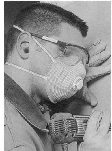
Figure 3.3.1.c. A double-strap respirator provides for a snug fit over the mouth and nose. If a respiratory protective device does not fit snugly, it cannot offer effective respiratory protection from small particles that can damage your lungs. A beard may cause the respirator to fit improperly.
