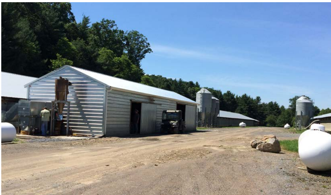
Figure 3. The Global Re-Fuel system at the Weaver farm is placed on a concrete pad between two poultry houses. The farmer needed to maintain the road between the houses, so the system was installed adjacent to one house and the ductwork to the other house was buried under the road.
