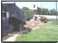
3 Dump parallel rows on base layer.
