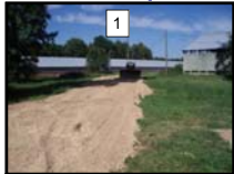
1 Bulking agent base -12 ft wide, 6-12 in. thick.
